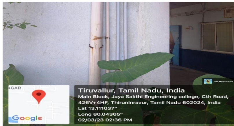
Rain water harvesting pit
