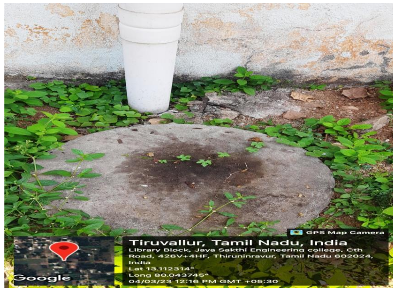
Rain Water Harvesting in Library Block
